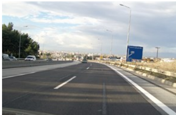
Highway A8 Olimpia Odos construction project in Greece uses the natural bitumen Selenizza
