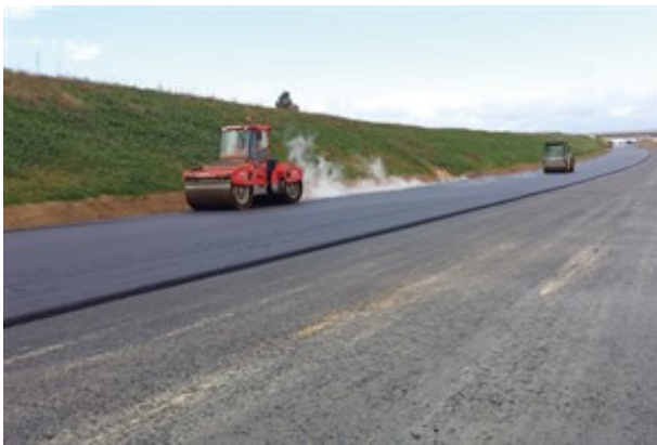
Highway A150 in France. An implementation of a two-layer pavement structure consisting of a 6cm HMAC wearing course and a 12cm HMA binder course, over a PF3 sub-grade
